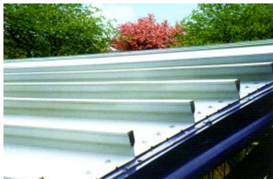
Structural liner tray on a new auditorium at Woldingham School. Surrey
